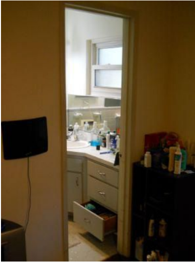
Master bath door missing
