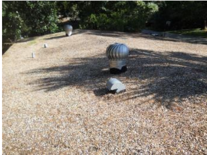
Gravel built up roof
