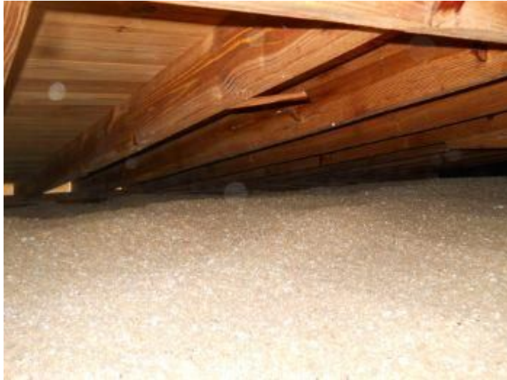
Insulation average depth 10-15 inches
