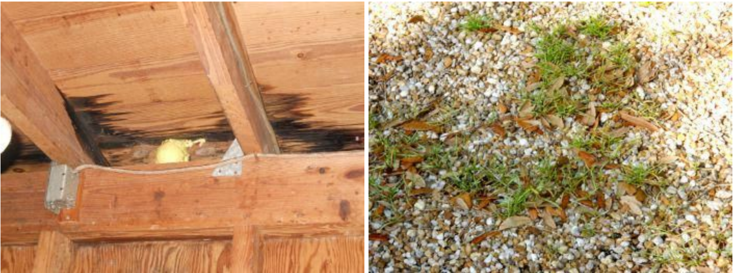
Sheathing moisture stains in utility room
